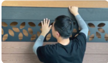
04 Step four Installation of lower tabs and fence panels.
