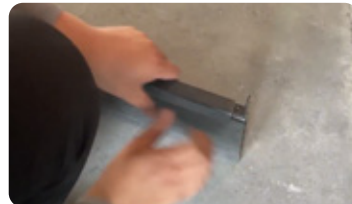
05 The fifth step Load the corner code on both sides of the upper clamping strip.
