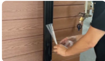
07 Step seven Tear off the aluminum alloy protective film
