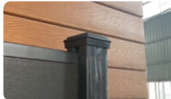
06 Step six Installation of column caps
