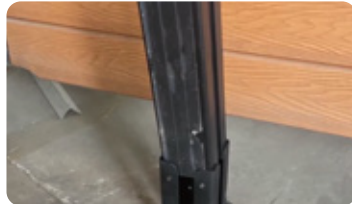
03 The third step Insert aluminum alloy column.
