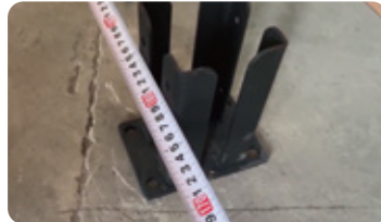
02 The second step Measurement of base intervals.
