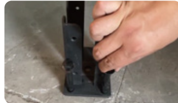
01 First step Drive in expansion screws.
